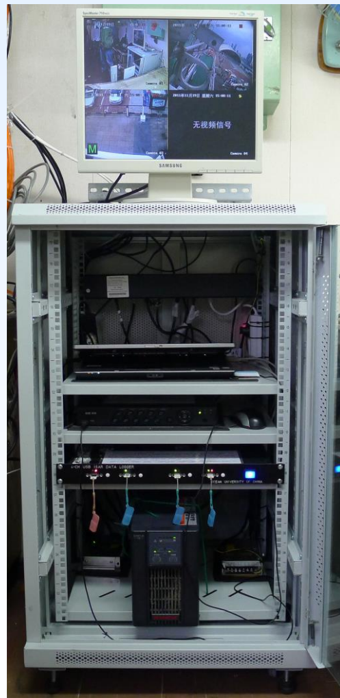
Data logging system in the lab
